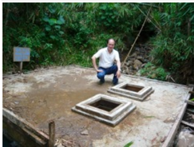
Spring water well just finished
