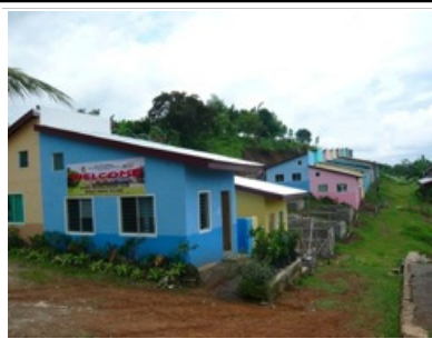
More houses being built on project site
